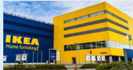
IKEA is all set to begin work of its biggest store in Noida
